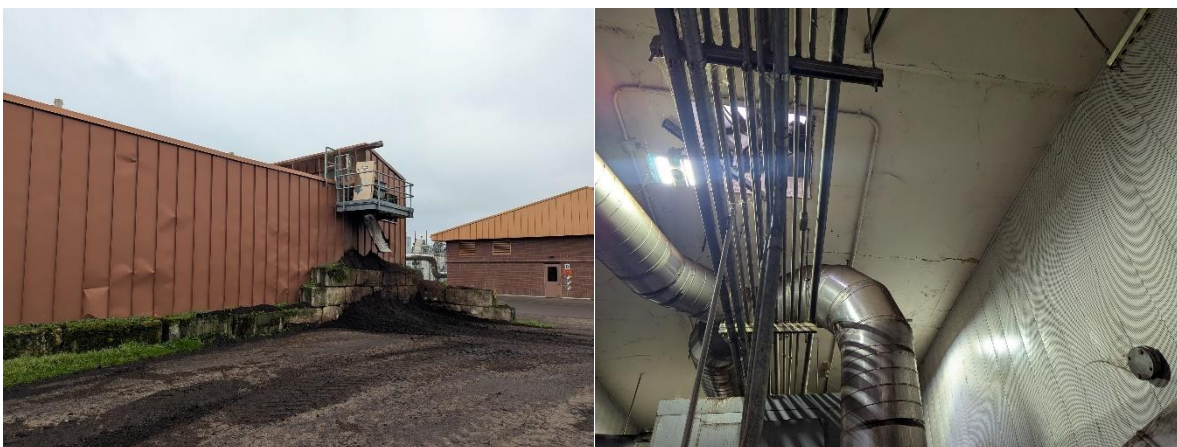
FIGURE 2-3: EXISTING COMPOST BUILDING
