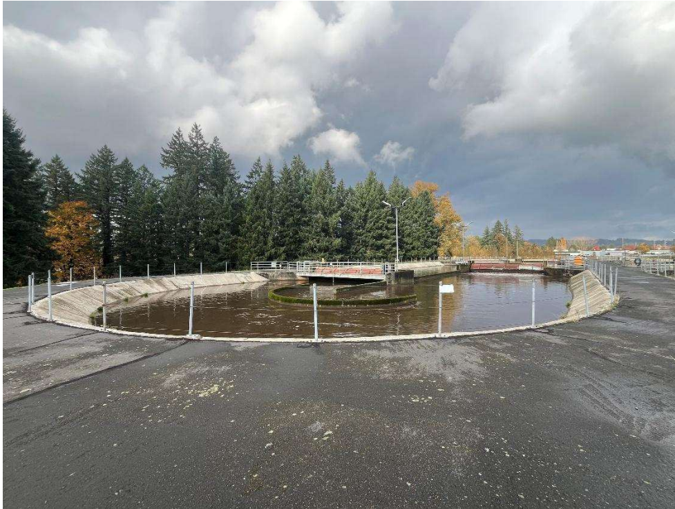
FIGURE 2-3: OXIDATION DITCH DURING STRESS TESTING
